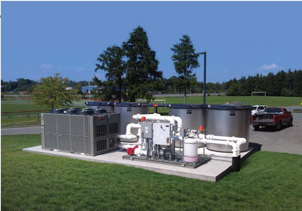
Skid mounted chiller plant - 200-ton peak cooling capacity with 90-ton, air-cooled, scroll chiller, pumps, controls and four ice thermal storage tanks
